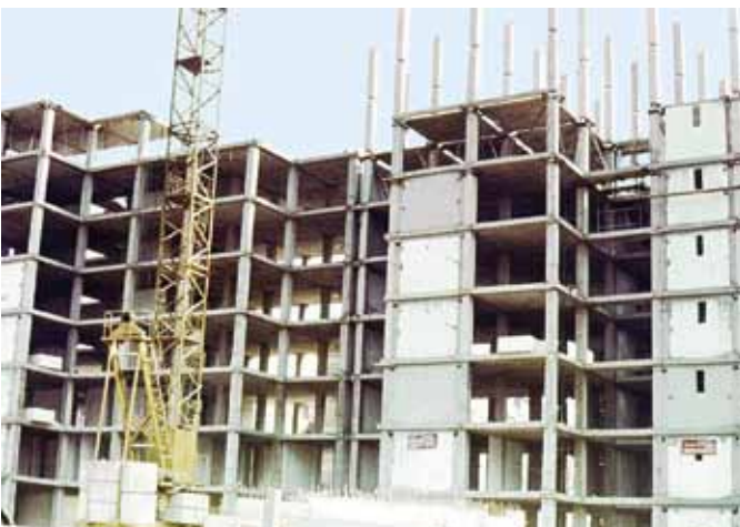
Figure 2. All-precaster concrete dual structure during erection.
